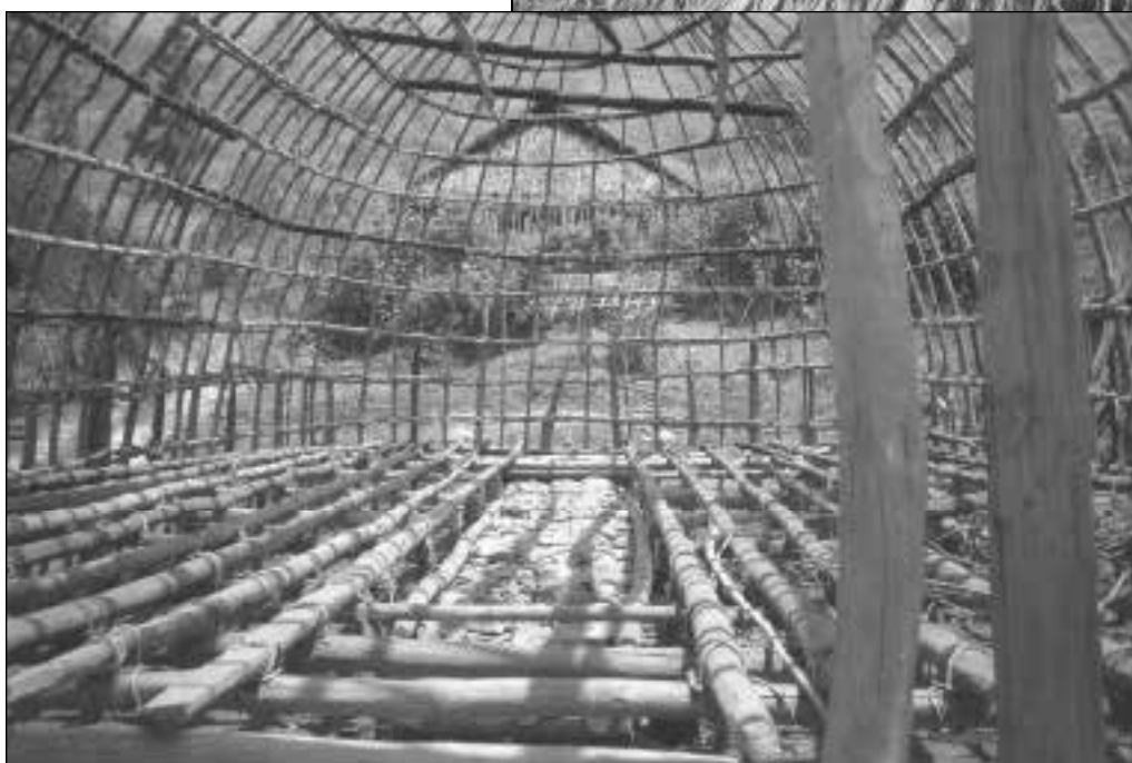
House being built - Nokopo (cliché C.K.Schmid)
