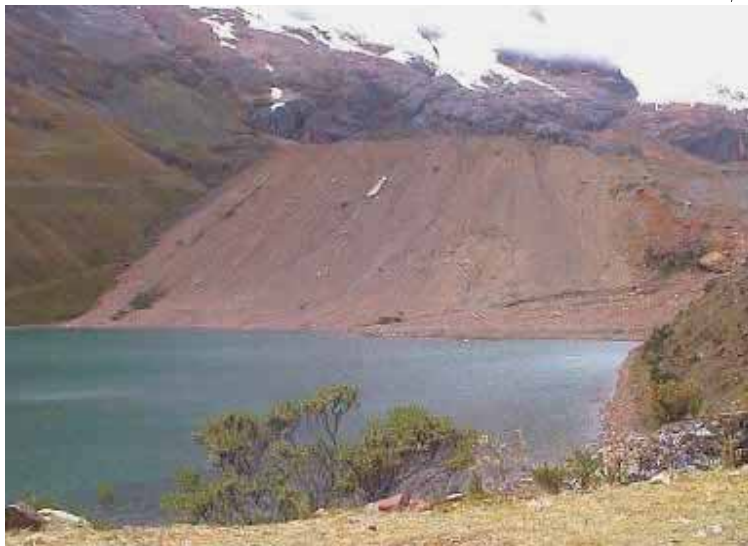
Safuna Baja and Safuna Alta moraine dam eroded by overflow
