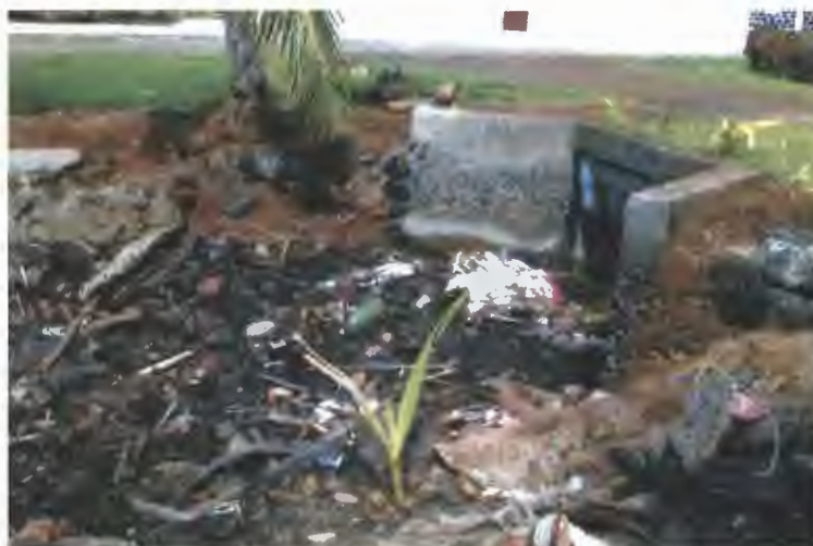
Figure 5 Wastewater outfall at Lalaleu.
