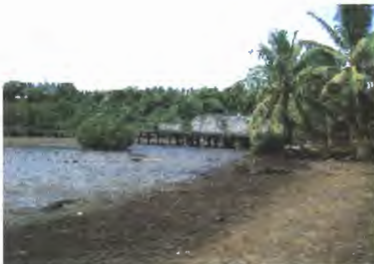
Figure 4 Coastal development - diverse construction activities within a mangrove forest.
