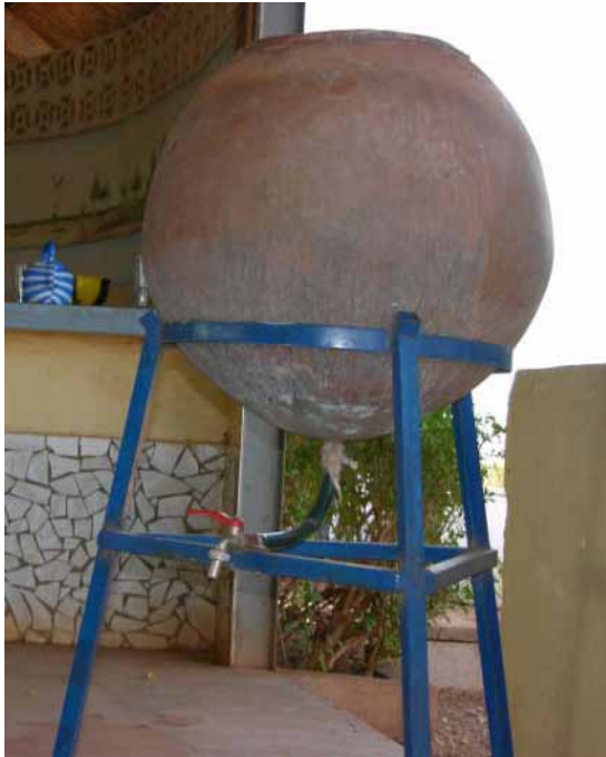
Figure 2. Safe water storage tank with simple tap in Kaya, Burkina Faso (Photo: Philippe Cecchi, December 2005)
