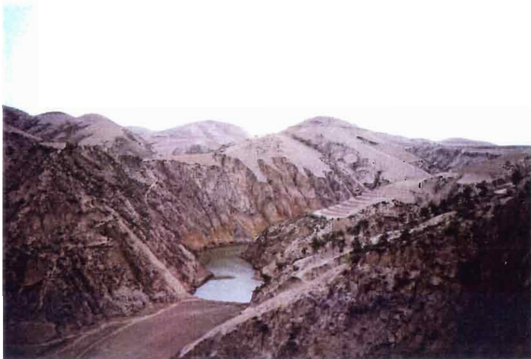
Photo 2 : silt-trap dam in JIUYUANGOU
