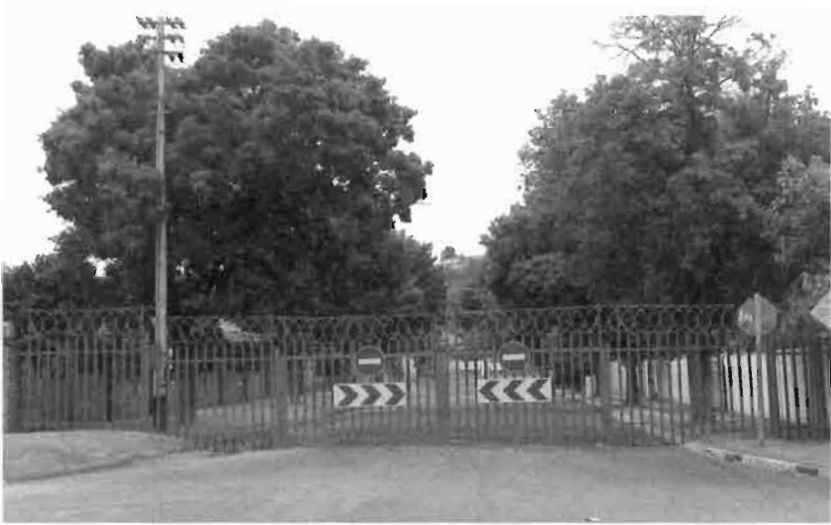
Fig. 2 – Closed public road with no entry signage
