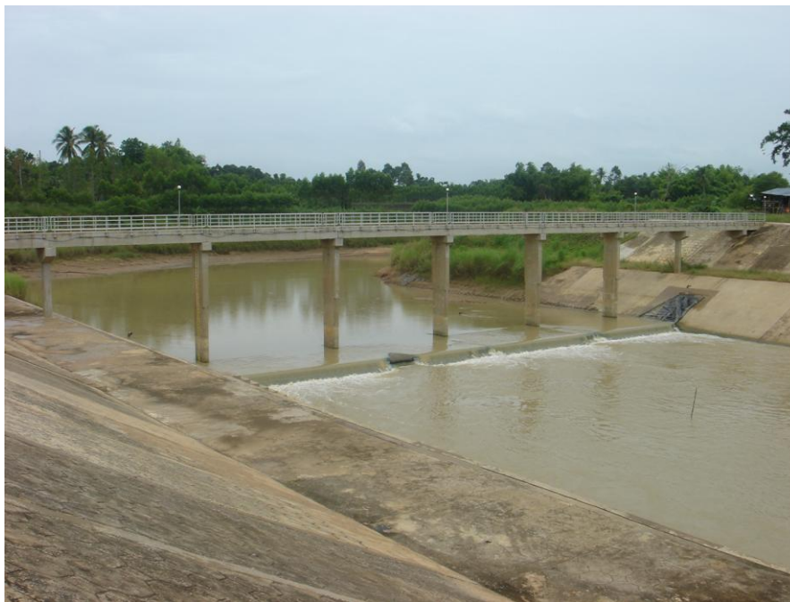
Figure 7. Rubber (inflatable) weir on the lower Phra Satung river
