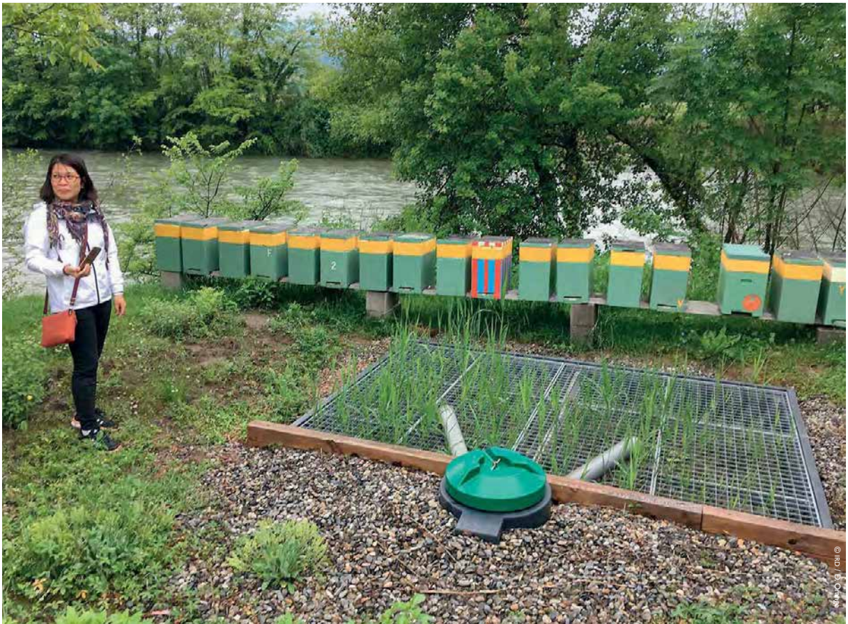
Example of a vertical planted filter for processing domestic waste water, with outflow directly into the river, France.
