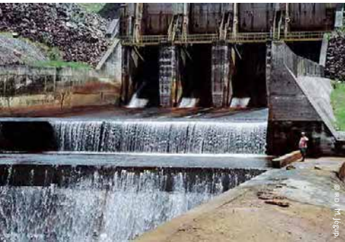
Rio Pitinga dam, Brazil.
