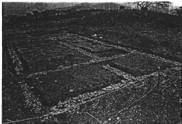
Figure 3. Multiroom, rectangular structure. A grass-covered roof could have been held by a wooden frame. The walls were probably made of adobe, thatch and daub, or both. The floor was a mixture of hard clay and tepetate.
