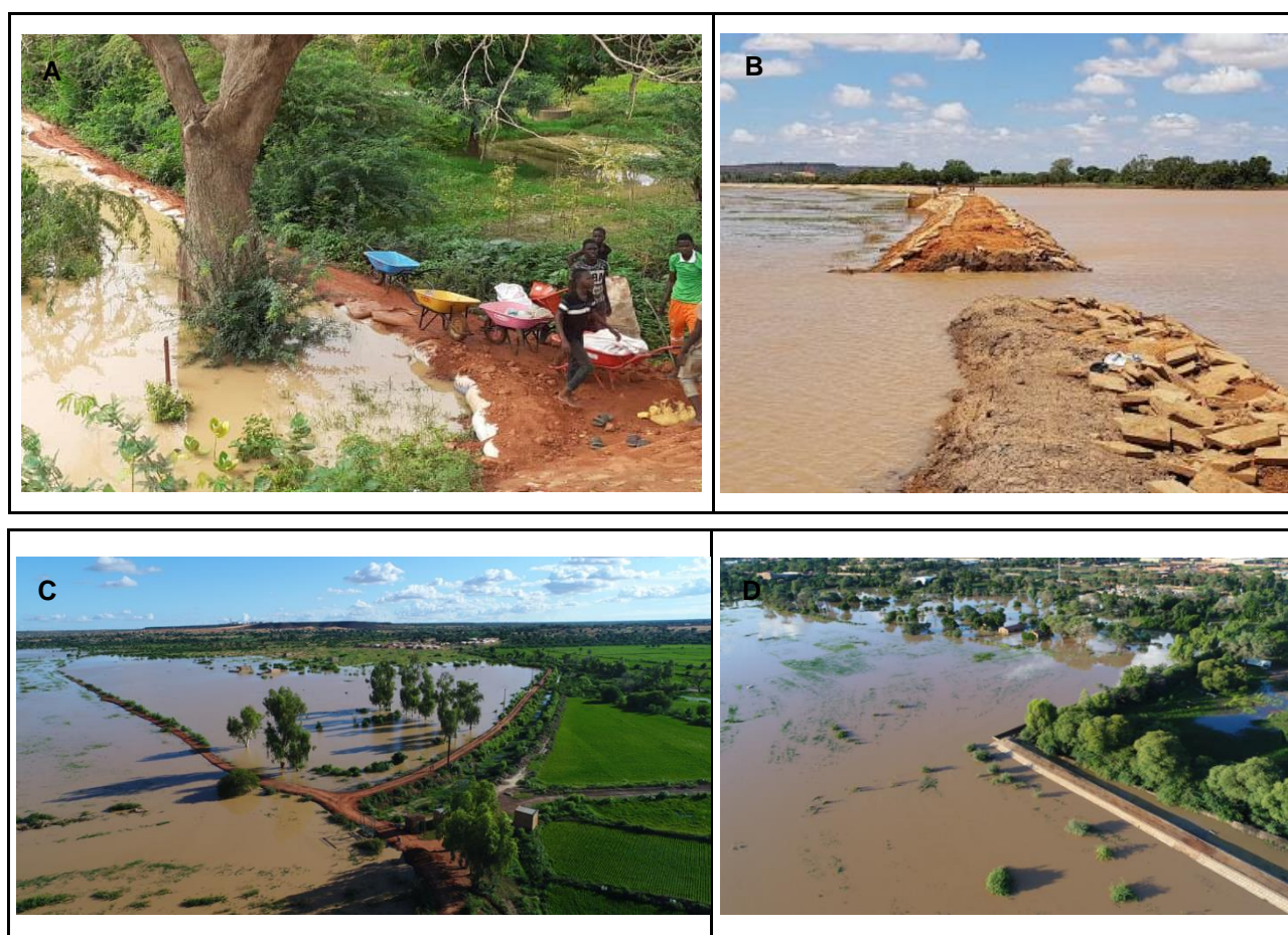
Figure 7. The Niamey levees during the 2019 and 2020 flood events: (A)(top-left) the bridges levee (sector B) raise with sandbags on 18/8/20 ( h = 651 cm), (B)(top-right) the levee break in Lamordé (Sector A) on 6/9/20 ( h = 679 cm), (C)(bottom-left) aerial view of Kirrissoie levee on 30/8/19 ( h = 619 cm), (D)(bottom-right) aerial view of Saga levee on 30/8/19 ( h = 619 cm).
