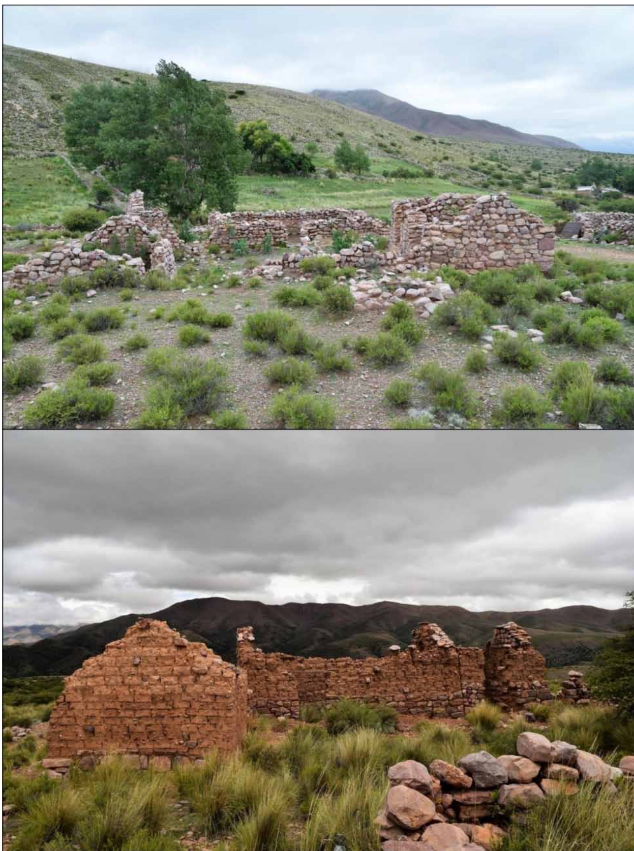
Figure 12. Abandoned houses in Rodero. The house above, built with stone walls, is older than the house below, with adobe walls (photo: Pablo Cruz, CONICET, 2019).
