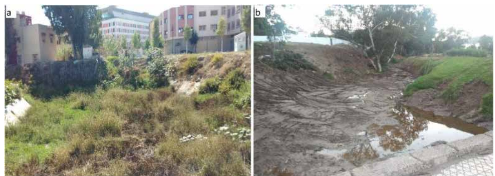
Figure 7. (a) Drainage channel not maintained or cleaned, (b) and drainage channel maintained and cleaned before the start of the rainy season (September 2021) in the city of Tangier.
