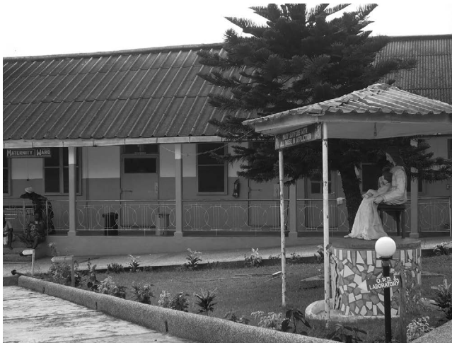
Figure 10.2 Public district mission hospital of Breman Asikuma in Ghana.
