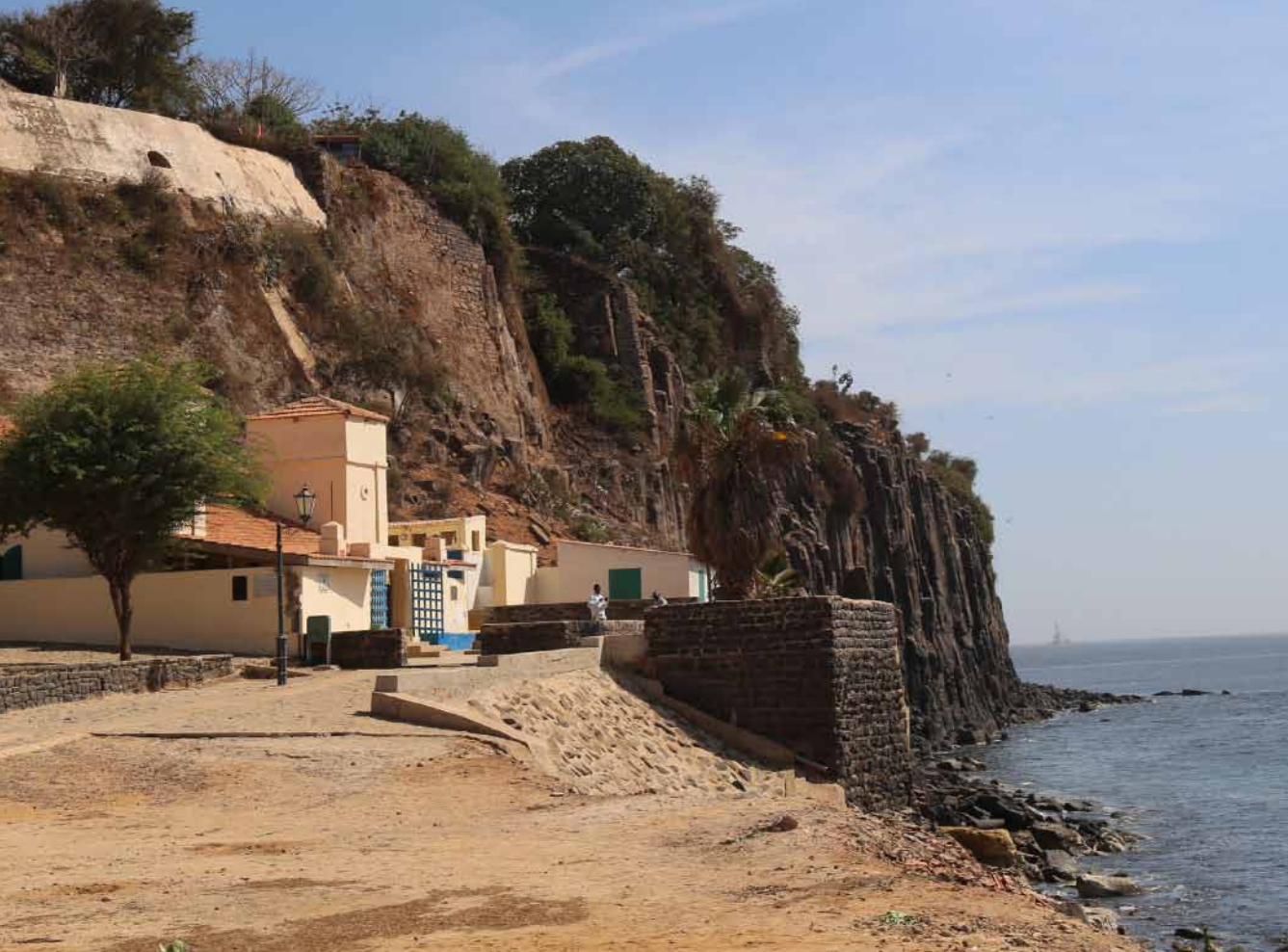
Cliff stabilisation in Gorée Island, Senegal. Photo: Madjiguene Seck/ World Bank
