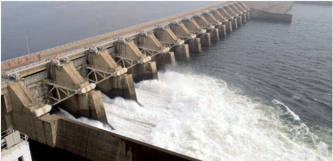
Kpong hydroelectric dam (Ghana).
