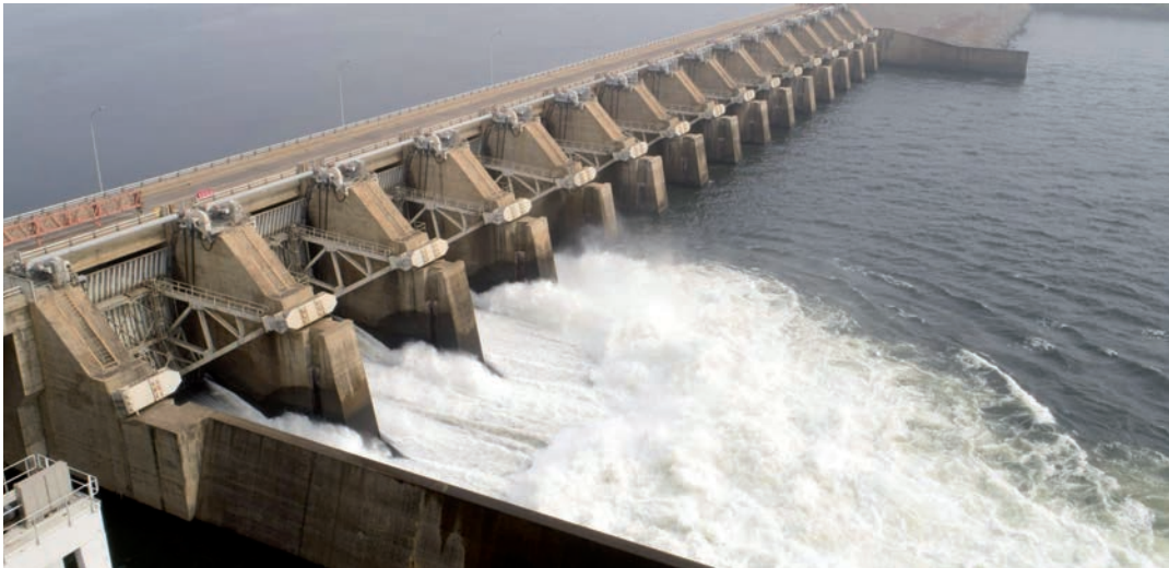
Kpong hydroelectric dam (Ghana).
