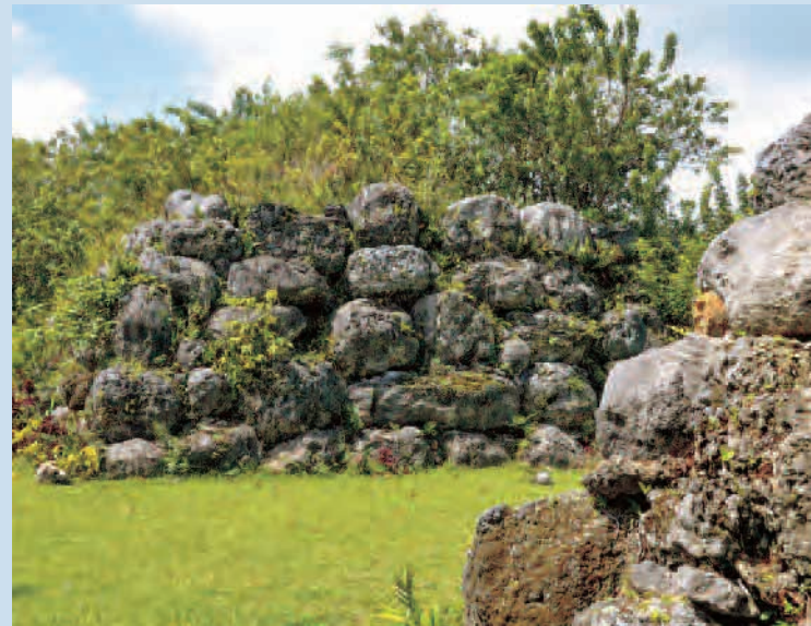
Monumental entrance to the megalithic fort of Hnakudotit, built on the Maré plateau using fossil coral blocks. © C. Sand
