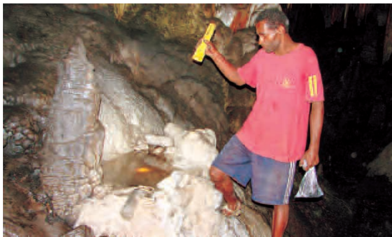
Artificial basin made of blocks of broken stalactites, built in a cave on the island of Tiga for the collection of infiltration water. © C. Sand
