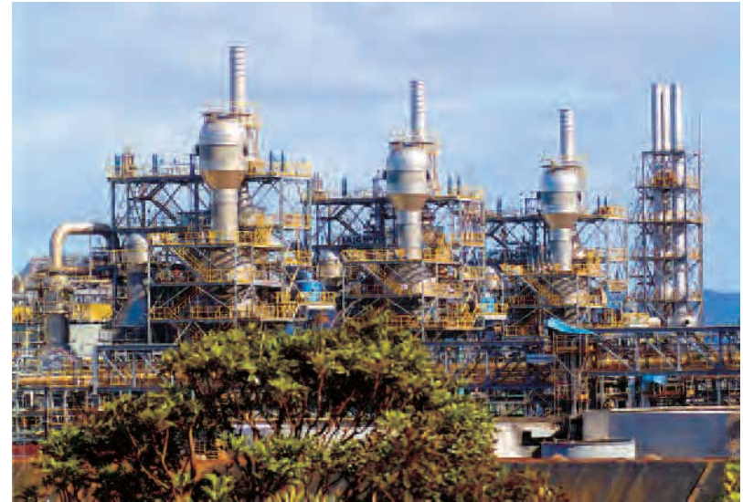
Mining processing plant, Vale, Prony. © P.-A. Pantz
