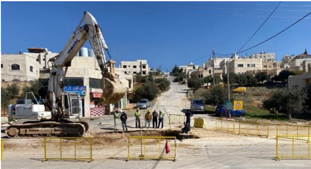
Building works on land purchased by a civil servants' cooperative in Amman, Jordan, 2021 © Kalaldehy
