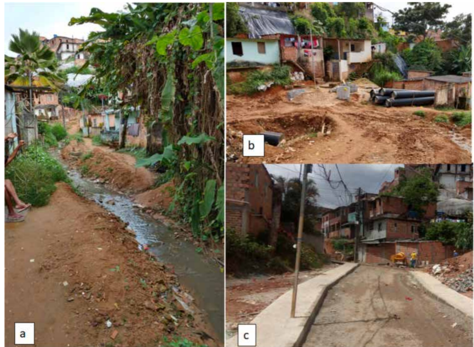
Fig. 1 Infrastructural intervention in Pau da Lima, Salvador-BA, Brazil; a typical open sewer in Pau da Lima, b cross-sectional area of an aspect of the community during the intervention, and c modification of sidewalks to reduce sewer water accumulation
