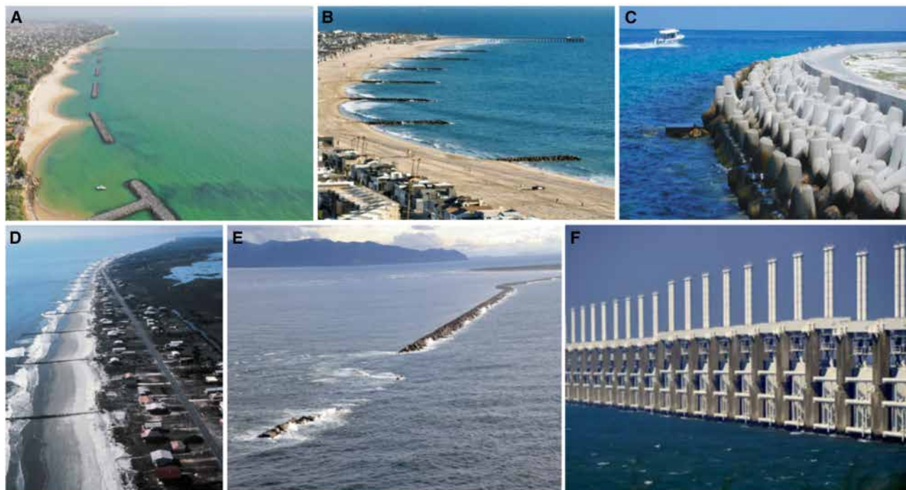
Figure 1. Coastal protection structures located around the globe
