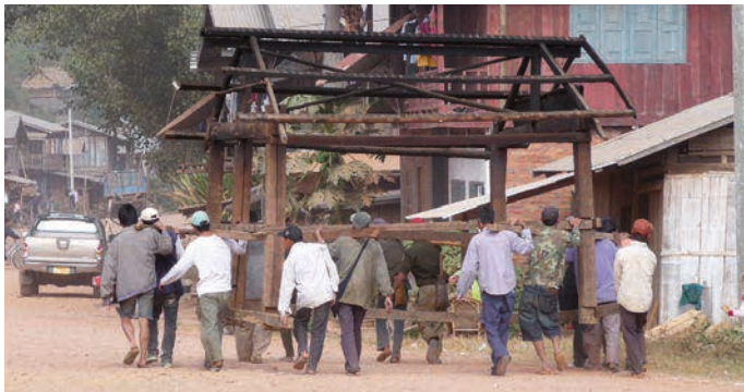
Moving. Relocation of a building structure
