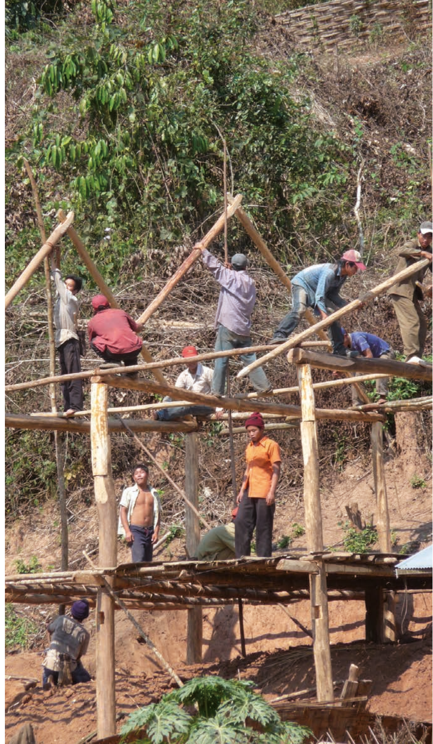
Construction of a house frame
