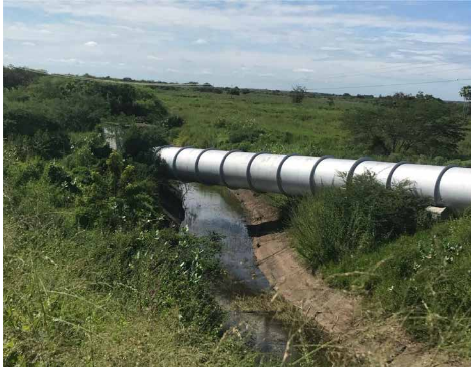
Fig. 2. Eixão Pipe crossing over PIMN Canal.
