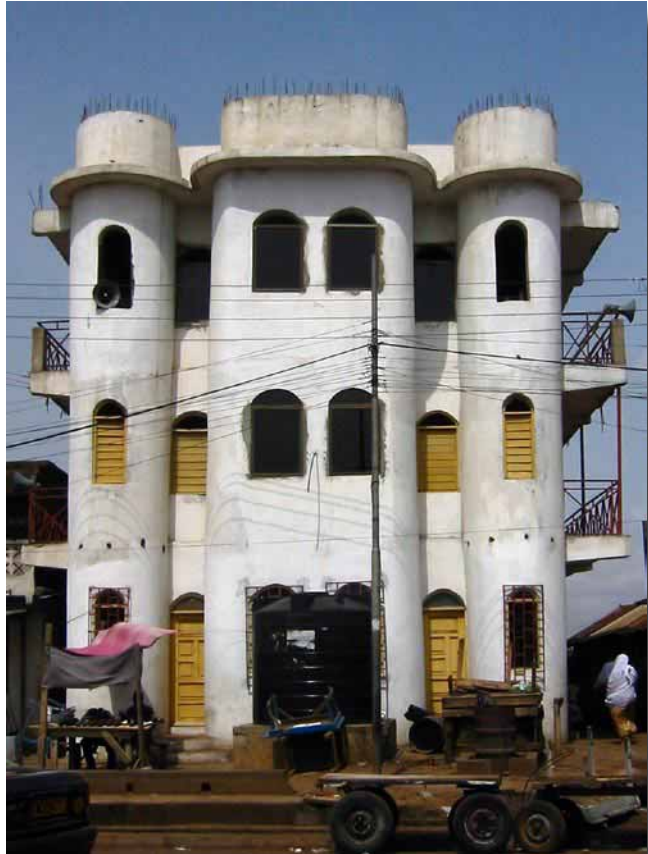
Mosque building in progress in an old migrant community in Accra
