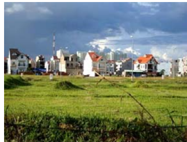
Ho Chi Minh City New housing estate in District 2 (PG, 2008)
