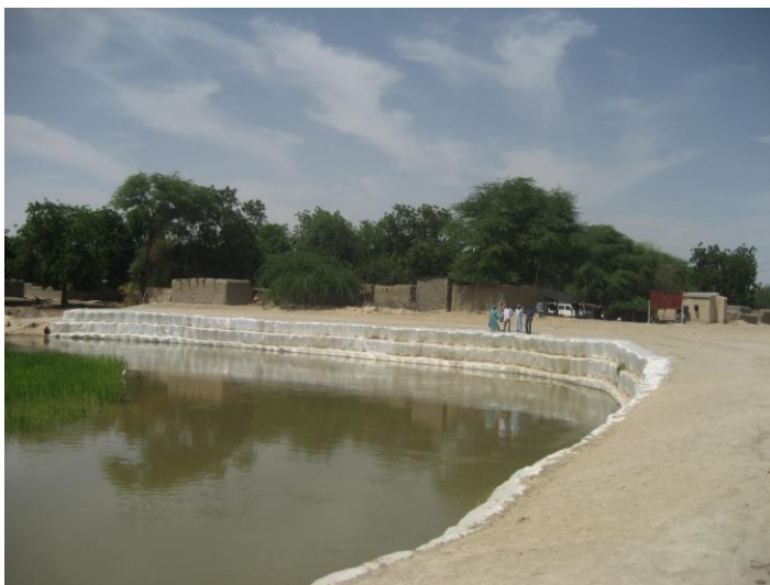
Figure 3.10. Reinforcement of the banks of the meander, by the local organization PADL, at Bosso.
