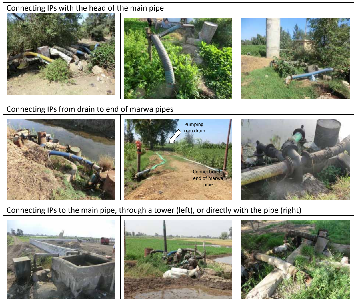
Figure 20. Connection of IPs to the distribution network
