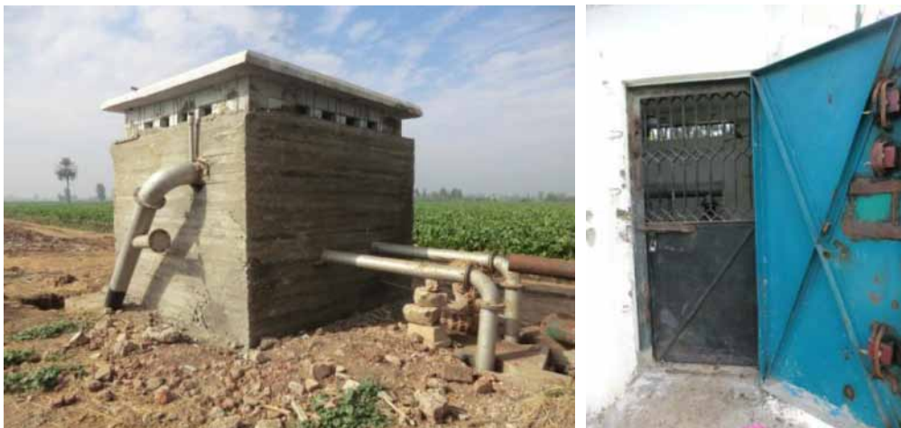
Figure 9. Pump station with a reinforced concrete protection
