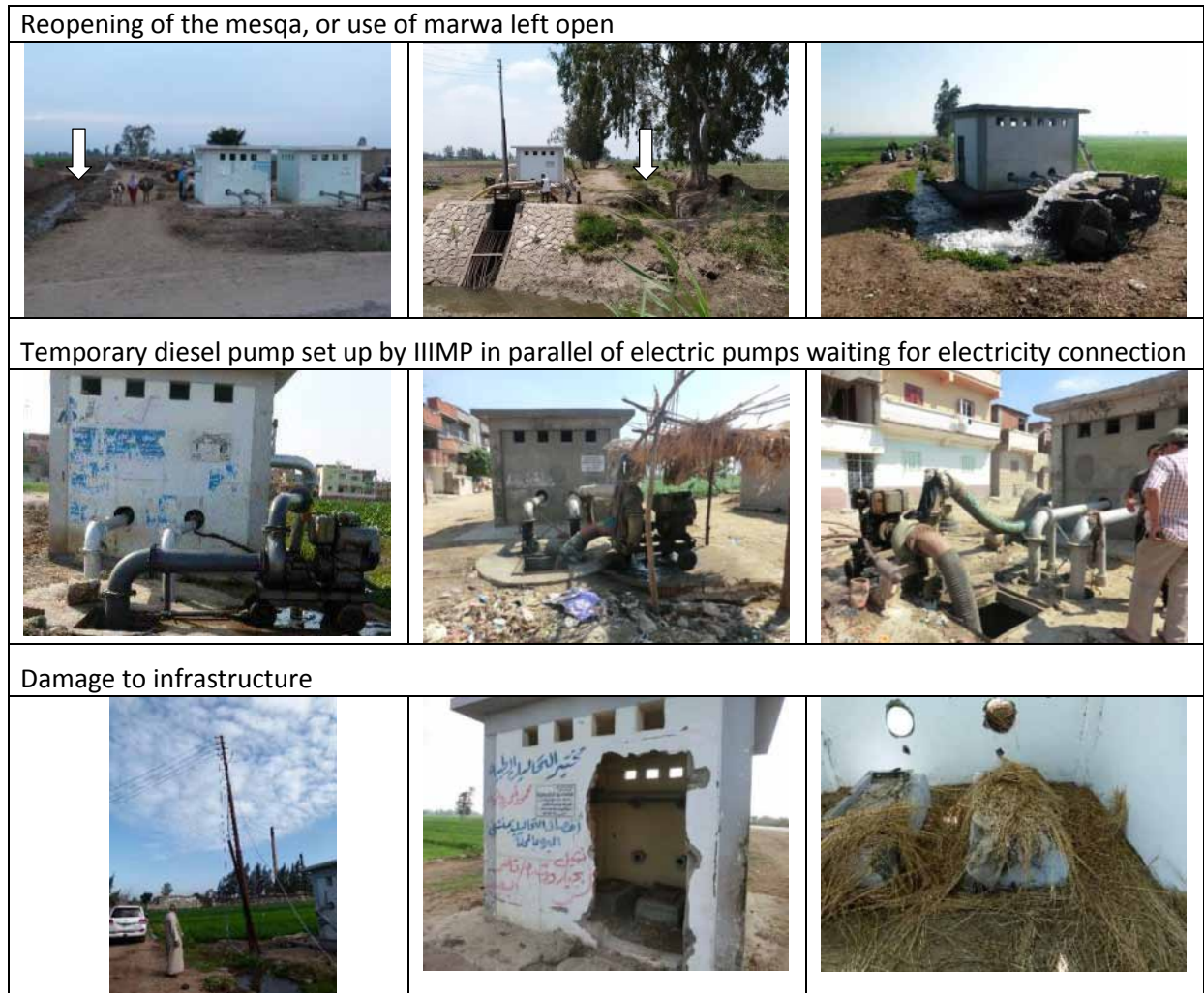
Figure 23. Consequences of delayed provision of electricity in IIIMP pumps
