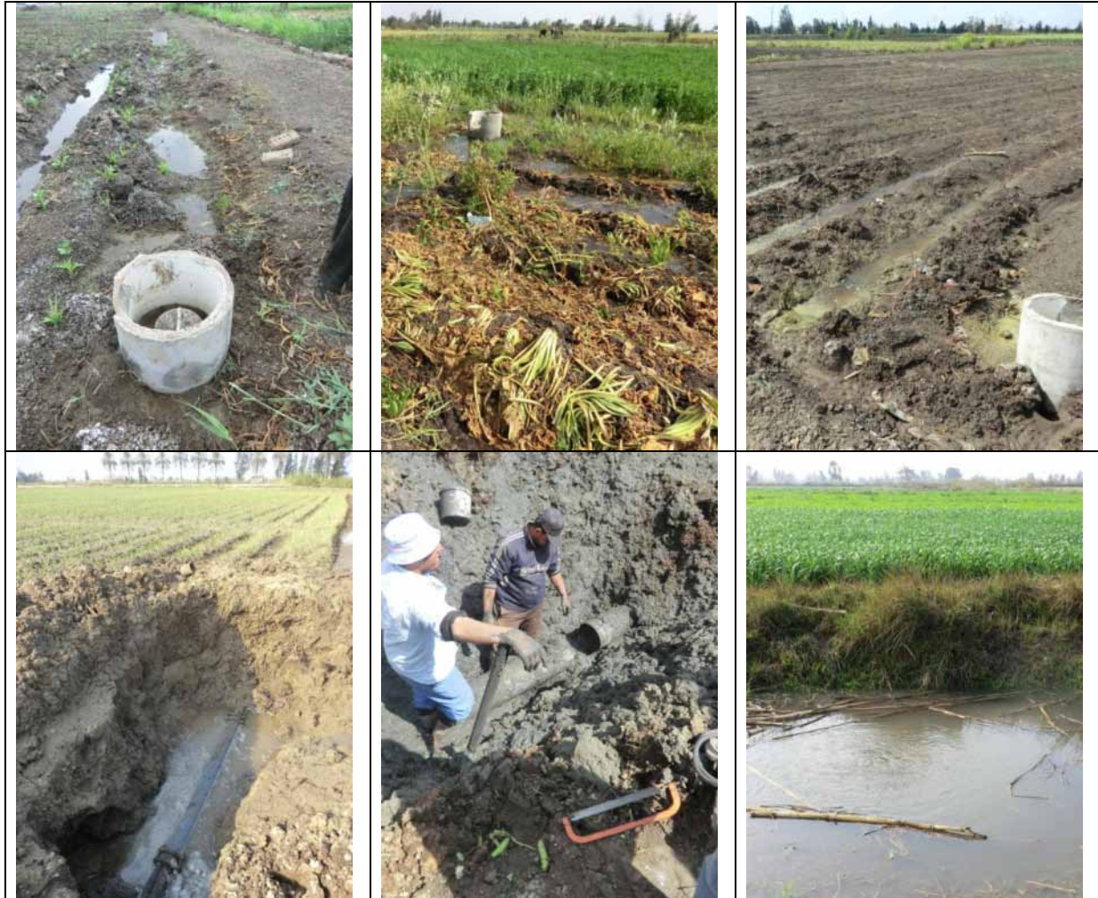
Figure 34. Seepage from buried marwa and mesqa pipes creating water logging
