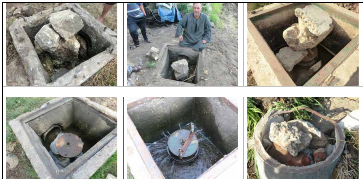
Figure 29. Problems of leakage with alfalfa valves
