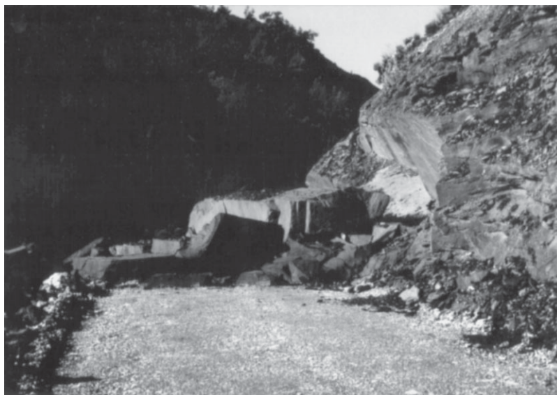
Figure 2. Blocks of fresh marl just after a collapse near Digne (Alpes de Haute-Provence, France), 1987. It is noticeable that rock fragments are not yet weathered and constitute solid blocks. Gravity remains the same; the excavation made for the road leads to collapse
