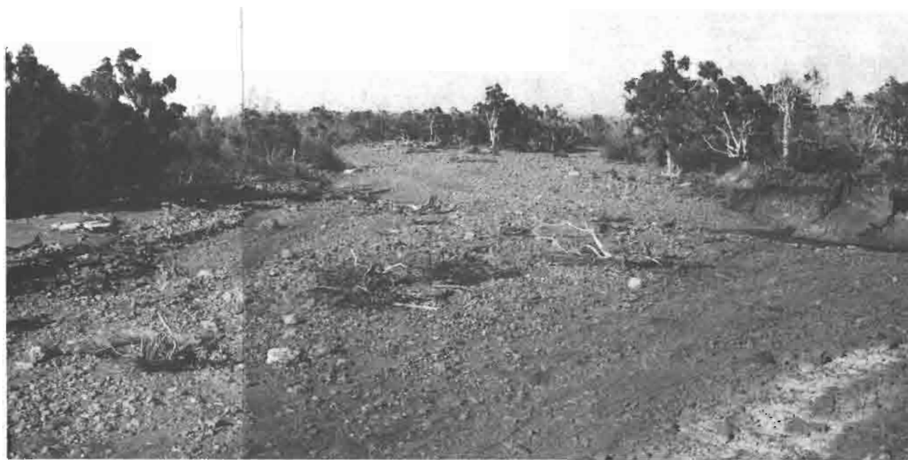
PLATE 6. The Oué Bouameu River Looking Downstream from the Highway Bridge. The channel was greatly widened and shallowed by accretion when floodwaters brought down large quantities of mining waste from the Kaala massif, drained by its headwaters. During Cyclone Gyan, in December 1981, large amounts of sand and gravel were swept down to the mouth of this river and deposited along the coastline at Karembe.
