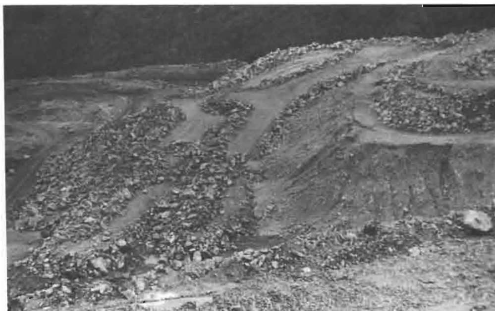
PLATE 29. Boulder Walls Built along the Contour on the Southern Slopes of the Thio Plateau to Intercept Downwashed Mining Waste and Reduce the Amount Discharged into the River Valley
