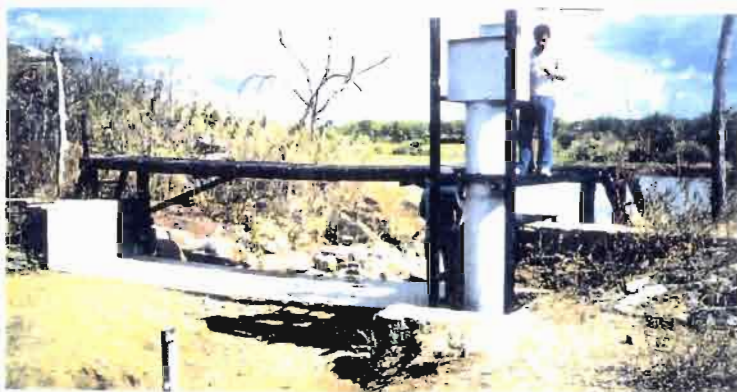
Station de Caldeirão
