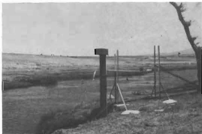
MALKA-WAKANA gauging station Station de MALKA-WAKANA
