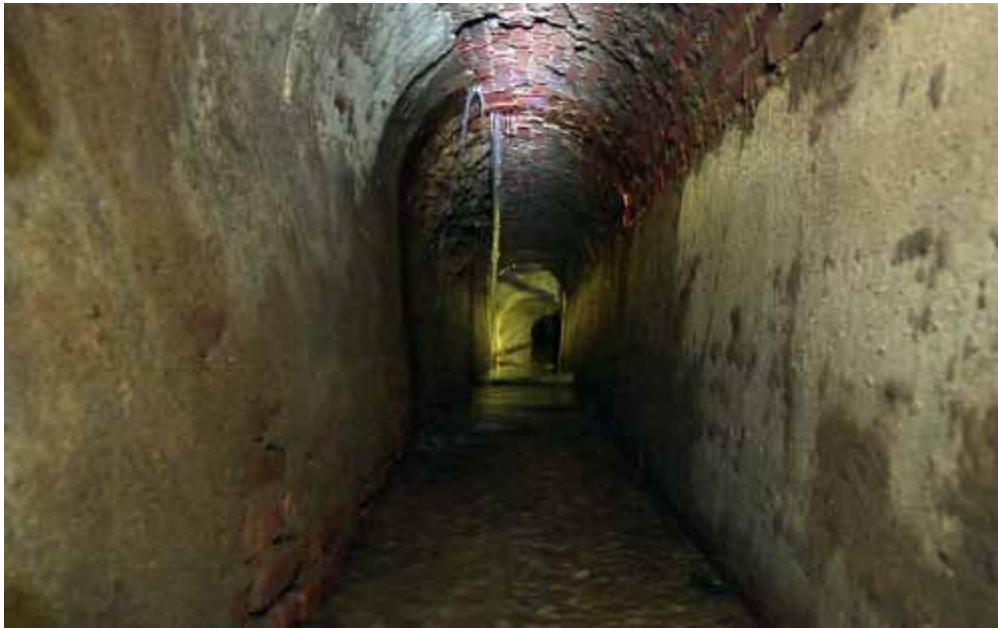
Figure 6: Deterioration of a French-era built sewer. (source: VNExpress).
