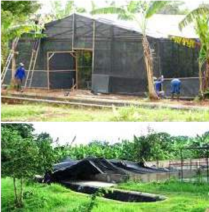
Figure 2-5 Above: original prototype of the insectarium in bamboo and fine wire mesh. Below: the same after violent winds
