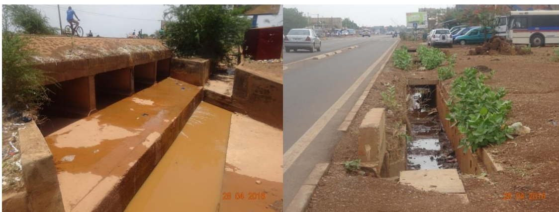
Figure 6. Open-air urban drainage channels in the city of Ouagadougou
