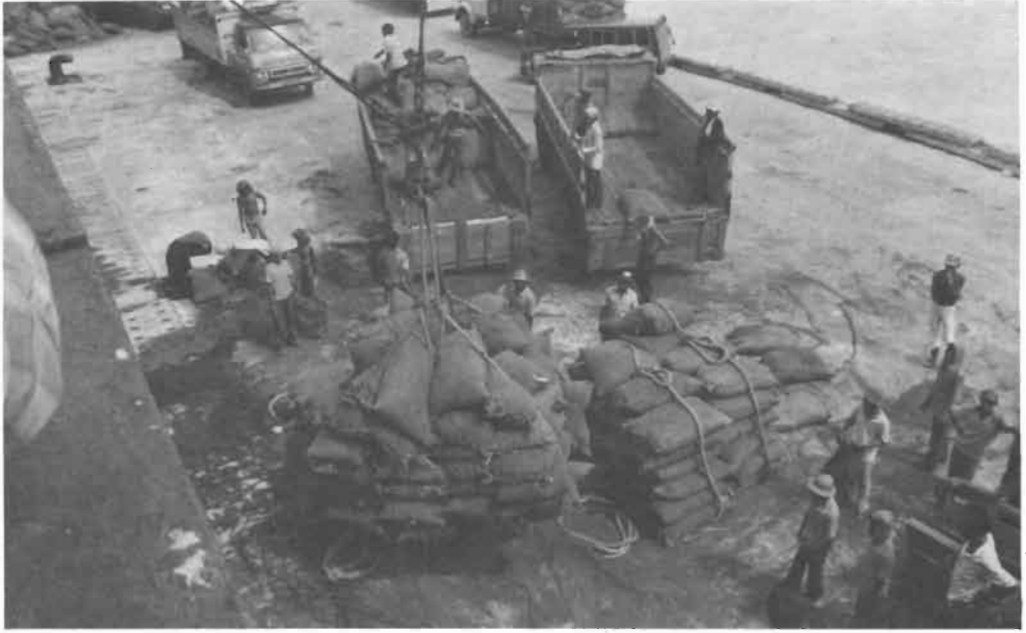
11. Insufficient harbor equipment leads to too many handling operations and increases the costs.
