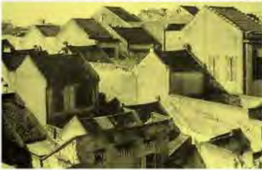
Old roofs (Hang Bac street, photo by Vo An Ninh, 1956)
