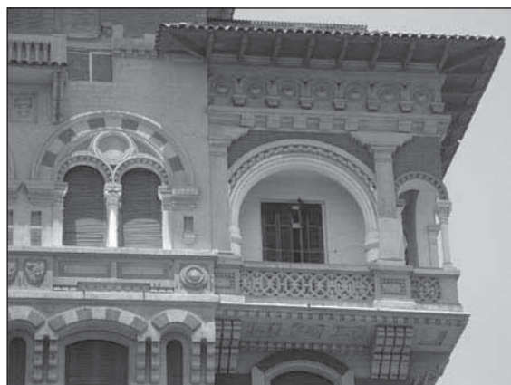
Fig. 3.20 Fine architectural details of buildings © ALEXMED
