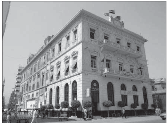
Fig. 2.53 The Municipal Council's headquarter, former casino, billiard room, meeting room, and theater, Al-Bahr St. © A. Bendary
