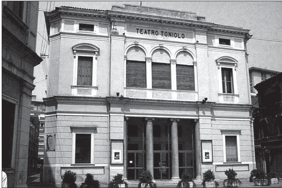
Fig. 3.33 Façade of Toniolo theater before works © Michielletto
