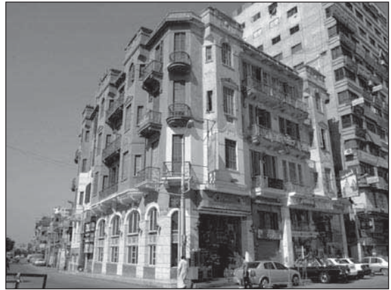
Fig. 2.52 Commercial Residential building, El-Thawra St. © A. Bendary
