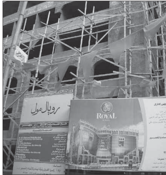
Fig. 3.21 New developments in the downtown area © Y. Aref
