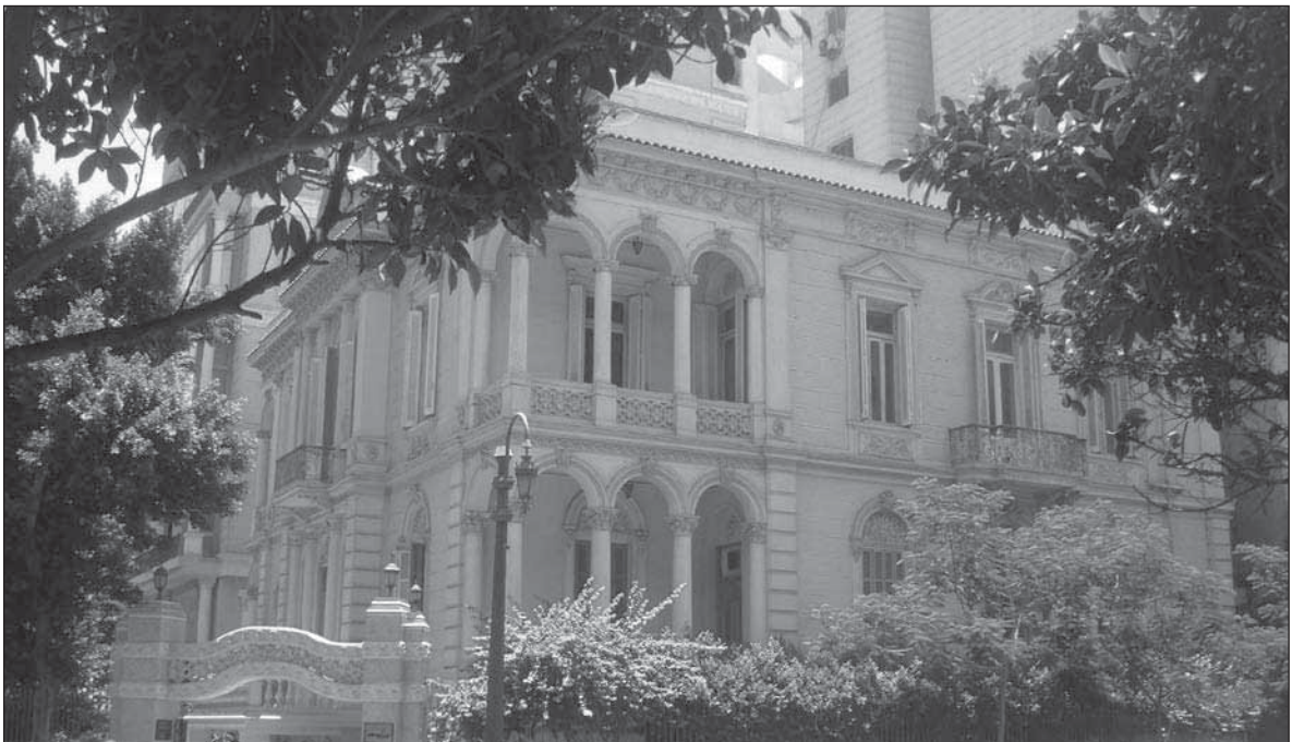
Fig 3.23 Rose El Youssef building, Down-town Cairo © S.Attia
