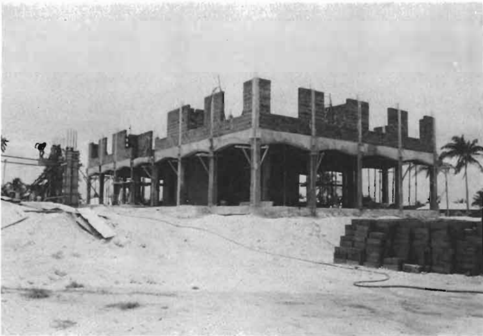
Fig. 7. Construction of the community shelter of ANAA atoll (Oct. 1984).
