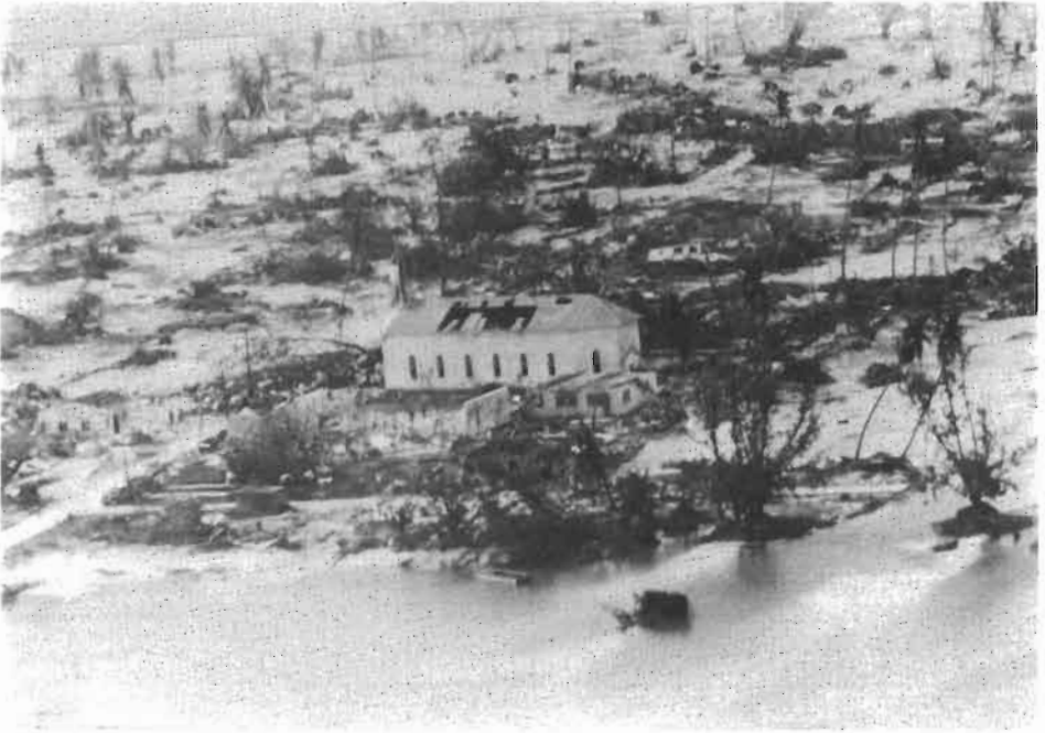
Fig. 3. The central part of the village of TUUHORA. ANAA atoll, after cyclone ORAMA. View taken from the lagoon. The storm surge came from the upper part of the photograph.
