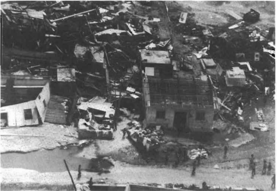
Fig. 4. The action of the sea on the buildings of TUUHORA. (Cyclone ORAMA). The storm surge came from the right.
