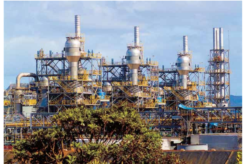
Usine Vale, Prony. © P.-A. Pantz
