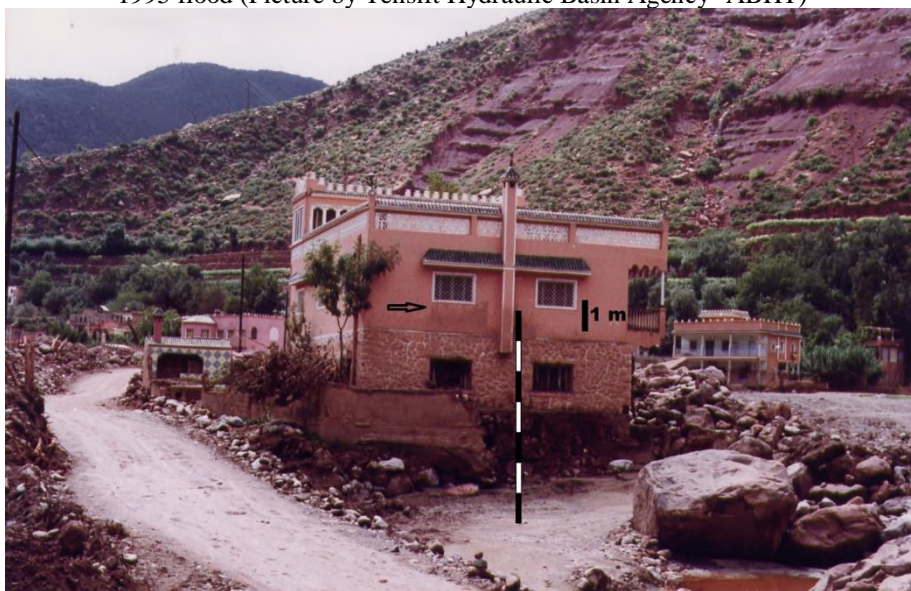
Figure 5: Other example of the water level reached during the 1995 flood
