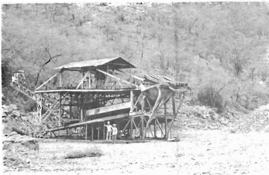
Figure 11. Dredge used in recent placer mining, San Antonio de la Huerta area.
