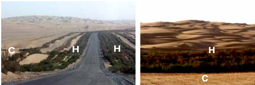
Figure 3.18. Wind erosion control methods to protect the road that crosses the 446 km of dunes of the Taklamakan Desert, Xinjiang, China: a strip of reed straw checkerboards (C), about 50 m wide, precedes at least six lines of hedges (H) irrigated from the water table and composed of several species adapted to desert conditions and salt water [CHE 15] (photos: C. Valentin). For a color version of this figure, see www.iste.co.uk/valentin/soils5.zip
