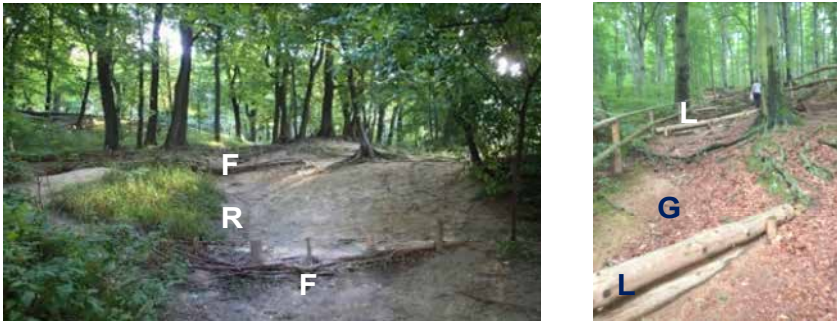
Figure 3.19. Methods to control concentrated erosion. On the left: a series of fascines (F) retain sediments from a channel (R), Zamok Park, Lviv, Ukraine. On the right: logs (L) were installed across a small rill (G) formed from a path in the beech forest, Chojnik, Poland (photos: C. Valentin). For a color version of this figure, see www.iste.co.uk/valentin/soils5.zip .
