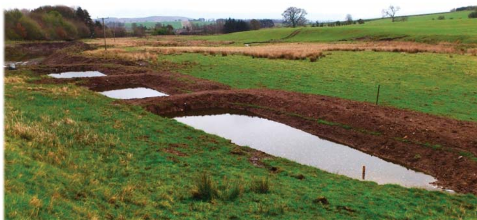
Figure 3. An example of a modified ditch with flow barriers acting as both a sediment trap and flood flow storage in Netherton Burn (photo from Barber 2013, credit to N. Barber).
