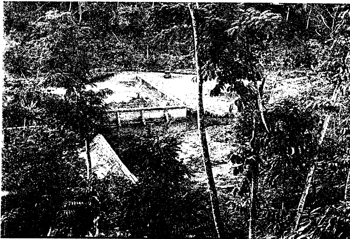
Headpond and flood spillway on VAISIGANO River
